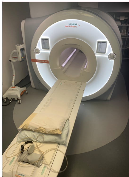
Figure 10. Example of change in floor colour to visually demarcate a specific threshold of the magnetic field.
