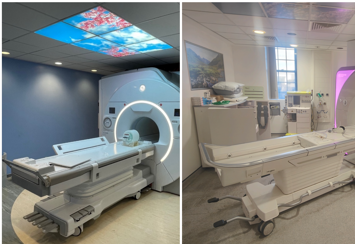
Figure 9. Example of artificial skylight designed for use in the MR Examination room and an RF-shielded window, both of which can help to improve the patient experience of an MRI scan.
