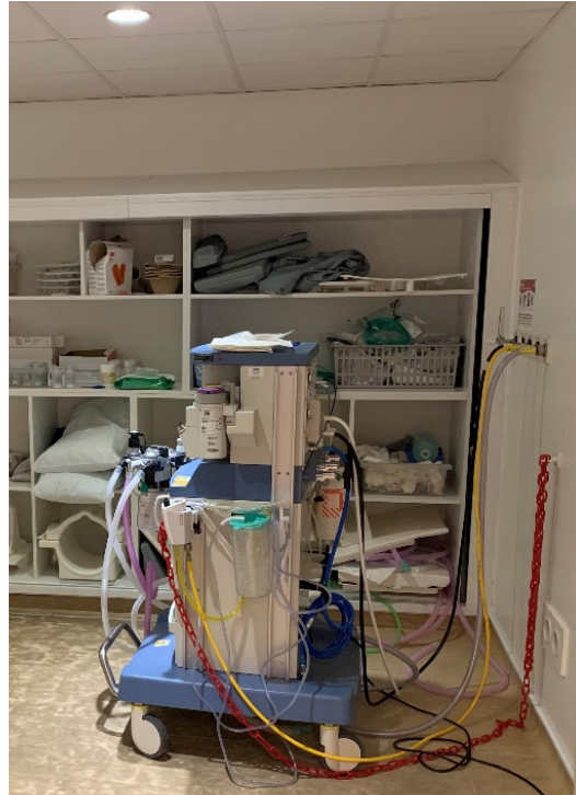
Figure 11. Example of anchor point in wall providing scope for non-ferromagnetic chain to tether an MR Conditional anaesthetic machine to avoid it being taken closer to the MR scanner than intended.
